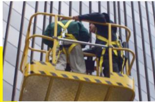
The ANSI standard for Boom-Supported Elevating Work Platforms (A92.5) and the Canadian standard for Boom-Supported Elevating Work Platforms (CSA B354.4) require that all personnel in the platform wear fall protection devices at all times.
